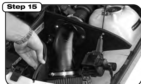
Place enclosed CARB E0 sticker on a clean/smooth surface on or near the intake system. E0 identification label is required in passing the Smog Check inspection. Your installation is now complete. Tighten all connections and clamps. Re-check after a few hours.
