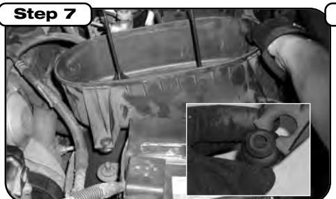
Remove lower half of air box. Remove rubber grommets from feet of the lower air box and save for use later. Remove filter minder indicator from factory air box for use later. Remove temperature sensor and save for use later.
