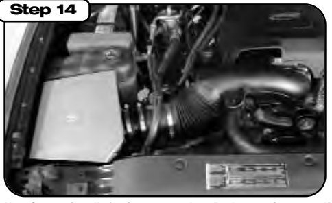
Step 14 Your Stage 1 installation is now complete. Replace engine cover. If installing Stage 2 Cx/Torque Booster Tube components, leave cover off. Make sure to tighten all clamps and check all electrical connections. Re-tighten clamps after a few hours of operation.
