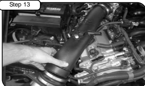
Step 13 Place couplers w/ Clamps provided onto both ends of intake and install new aFe intake tube. Tighten clamps with 5/16 or slotted screwdriver. Re- install Factory crank case breather onto new aFe intake tube.
