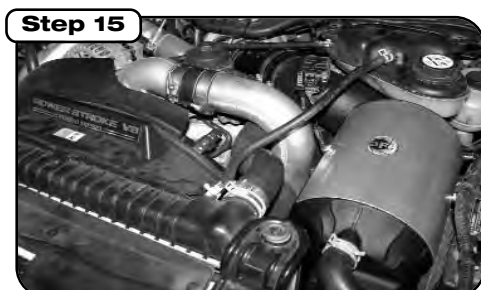
Step 15 Complete intake installed. Make sure all clamps are tight and that all electrical components are secure. Check and retighten connections and filter after a few hours of operation. Reconnect battery terminal. Thank you for choosing aFe!
