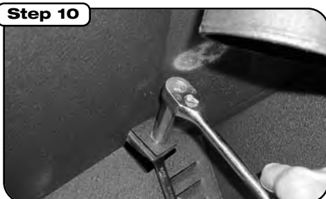
Step 10 Using provided bolts, locking nuts and washers on both sides of the bolt, fasten lower tab on heat shield and slotted hole to the existing rubber mounts. Be careful not to over-tighten, it is only necessary that the rubber mounts be slightly compressed. Fully tighten shroud.
