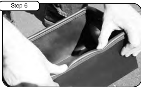
Install 7/16" trim seal to housing.
