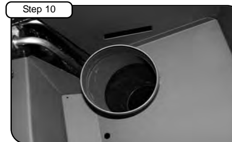
Position housing onto reducer coupler.
