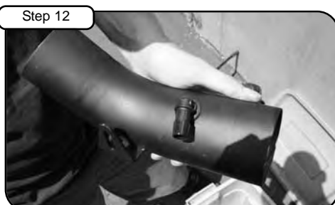
Step 12 Install 1/2" fitting in grommet.
