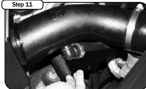
Step 11 Now that your hole is drilled re-install the aFe intake tube and insert the elbow. Your installation is now complete. Make sure you tighten all clamps and check all electrical connections. Re-check periodically.
