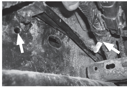
Image shows lines clear on the frame opening it up for the brace installation.
