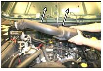
**2.** Remove the intake tube and resonator from the vehicle.
