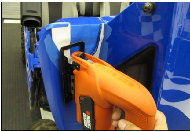
7. Using a jig saw or equivalent, follow the template and cut out the Duct relief.
