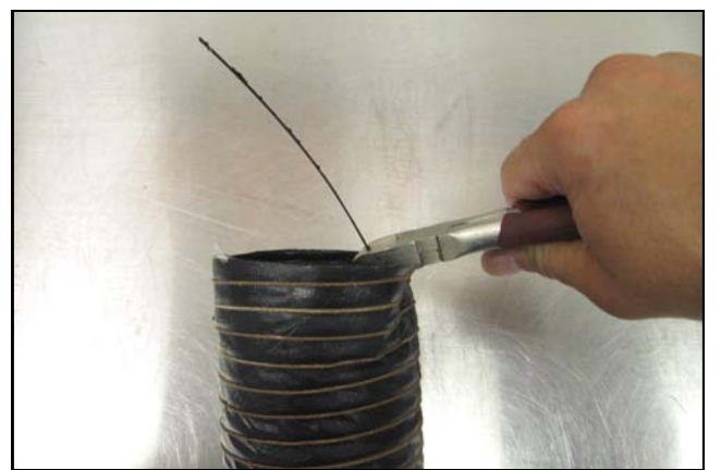
9. Using a pair of dykes, pull out approximately three windings of the steel wire inside of the Ducting (#6) and cut it off.
