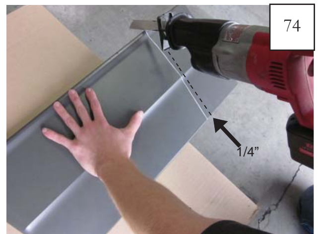
Using a reciprocating saw or other suitable tool, cut the factory side cladding approximately 1/4" back from the line drawn in step 70.
