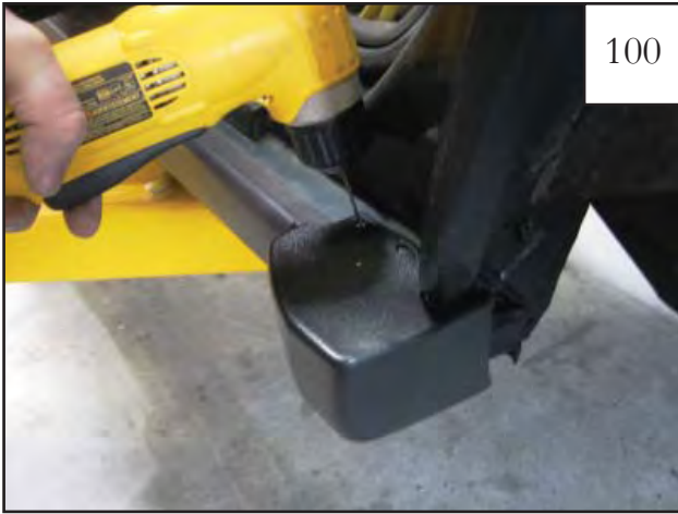
Drill marked holes with 3/32" drill bit.
