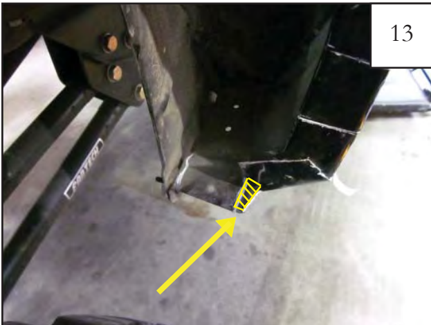
Using a Sawsall, cut off outlined area.
