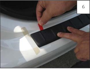
Maintaining part placement, repeat process for red tab liner nearest the front of the vehicle.
