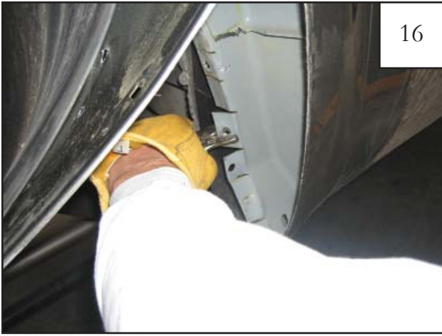
Bend lip straight with pliers between cuts made in previous step. NOTE: In Step 20, existing cuts will be extended after reference lines are marked.
