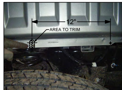
Figure 10.1: Inside Driver Side Rear Wheel Well
