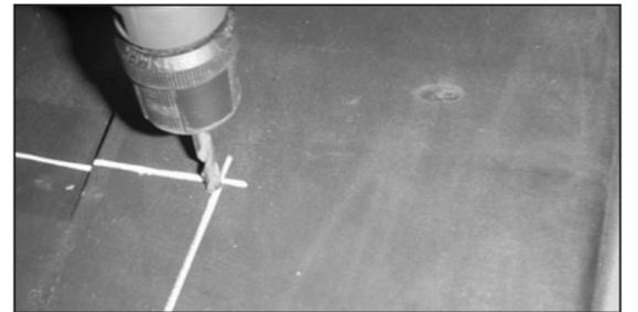
45. Using a 5/16" drill bit, drill a hole where the horizontal and vertical lines intersect.
