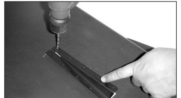
47. Hold the right angled "Z" bracket in place, using a 3/16" drill bit, drill out the five outer holes.
