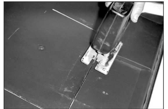
46. Using a jigsaw, cut along the horizontal and vertical lines. **Note: It will be necessary to clean up the cuts with a file.**
