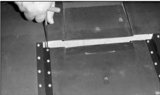
51. Secure the flap to the brackets with the hardware provided.
