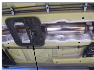
TUNNEL BRACE (TO BE RE-USED)
