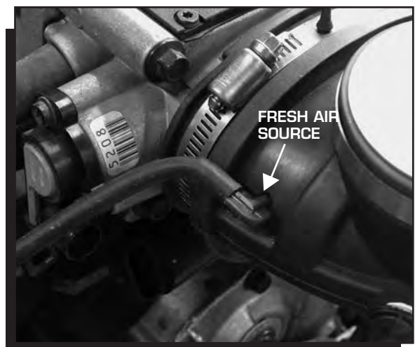
Figure 9 Installing the Fresh Air Line.
