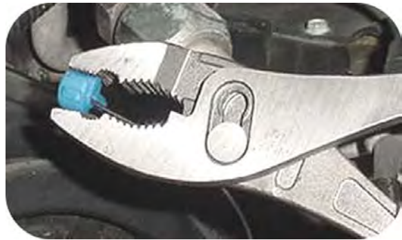
Figure 4 (Close T-Tap connector)
