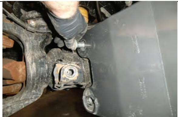
Stage 2 Install new assembled radius arm w/ OE bolts at top
