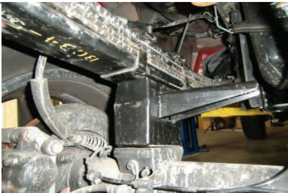
Place new lift block into original position and raise axle
