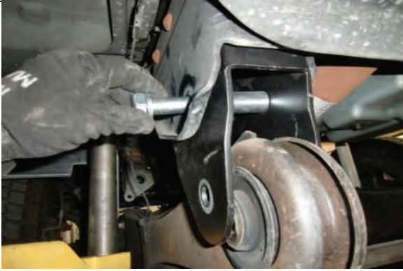
Stage 1 Install new radius arm drop brackets
