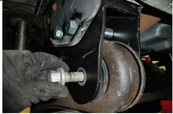
Stage 1 Raise radius arms and reattach to drop brackets
