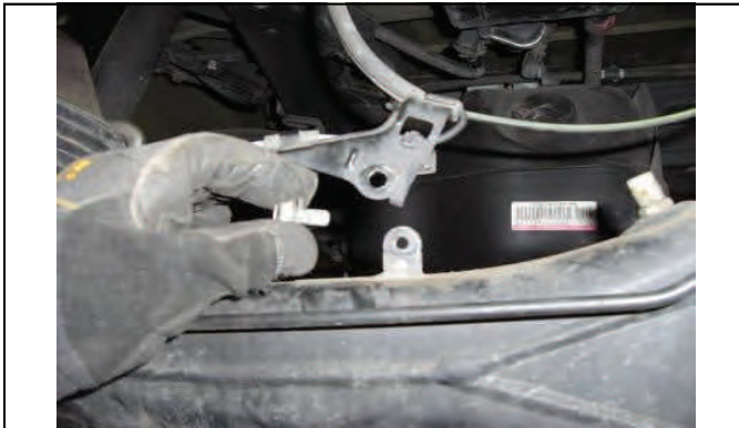
Disconnect ABS wiring brackets from axle.
