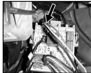
Electric Junction Box with Adapter Connected
