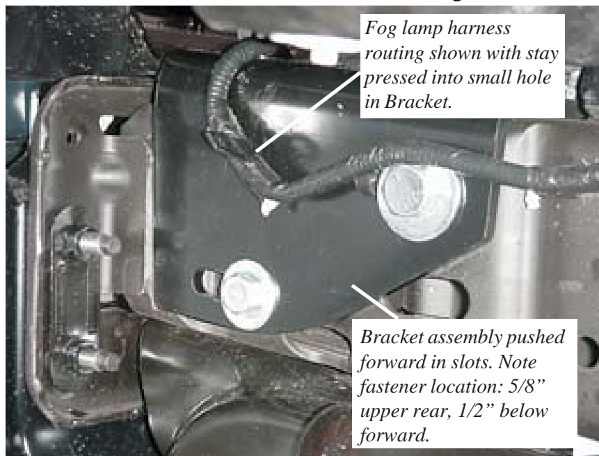
Figure 4 - LH Bracket Assembly Installed
