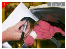
(Fig. D) Next using the template as a guide mark using a sharpie or scribe as shown above.
