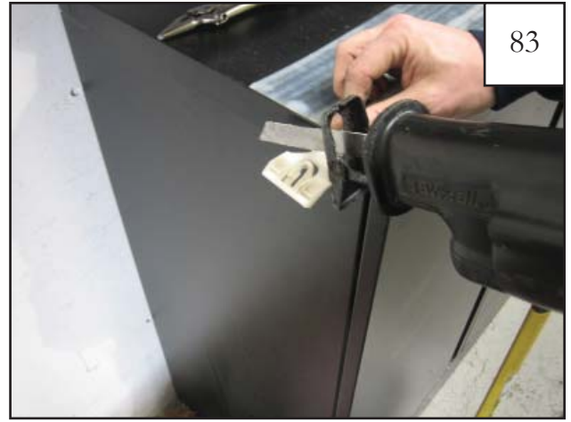
Using a reciprocating saw, cut the cladding clip just below the top section.
