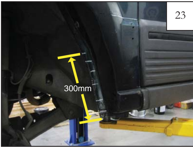
23 Mark fender flange 300mm up from crease of pinch weld. Mark horizontal lines below 300mm mark in between the spot welds on the pinch weld.
