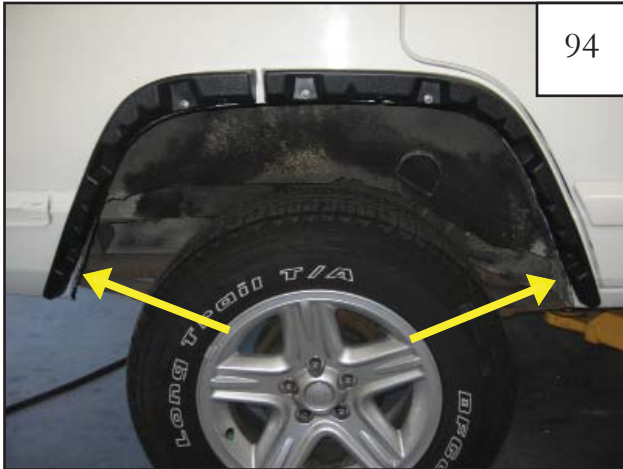
Install tuflocks in two lowest hole locations on inner pieces P3 & P4 (D3 & D4 for driver's side).
