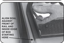
B. Peel paper back, align and adhere Element Seal<sup>TM</sup> at one corner across box to opposite corner and cut to length.
