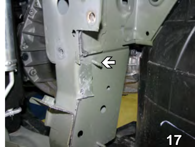
17. On the driver's side, using the reciprocating saw, cut off the bolt which was behind the piece removed in step 15. Flatten all sections flush against the frame rail with hammer.
