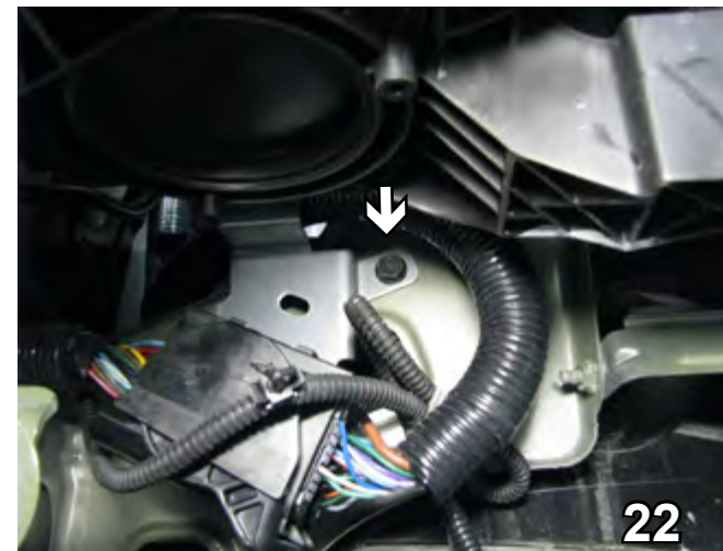
22. On the driver's side, use the 10mm socket to remove the screw holding the electrical box mechanism. Move the screw up higher out of the way of drilling and reattach.
