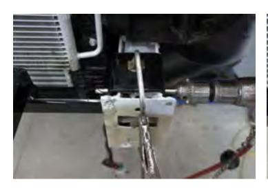
13. Drill the top front hole thru frame using a 13/32" drill bit. DO NOT drill remaining holes at this time.
