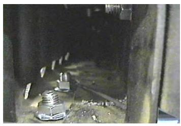
Using the base plate as a template, drill the remaining hole, with the 17/32" drill bit, on frame bottom, each side. Install items 2, 3, and 4 into place, refer to drawing on last page. Be sure and use loctite on all bolts before tightening.
