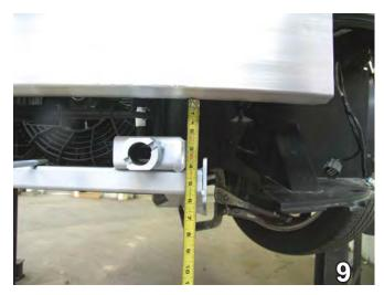
Align the baseplate against the lower frame extensions, so that the top of the crosstube is four inches from the bottom of the bumper. Clamp the baseplate in place with the large vise grips. Baseplate is painted white for illustration only. Actual baseplate is black powder coat.
