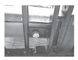
9. Drill holes for bottom of metal bumper, use baseplate as a template.
