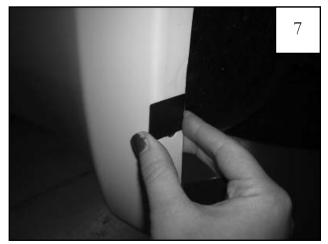
Remove flare and center a Tab (MT1-0002) over each of the four locations marked in Step 5.
