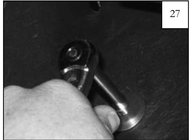
Install a supplied SS Fender Washer (WA1-0015) and supplied 5/16" Nylock Nut (NU1-0019) on back of screws installed in step 26 and tighten. (Note: Tighten from the back )
