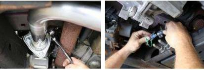
**13.** Now, install all (4) O2 sensors in the proper location, be careful not to damage.
