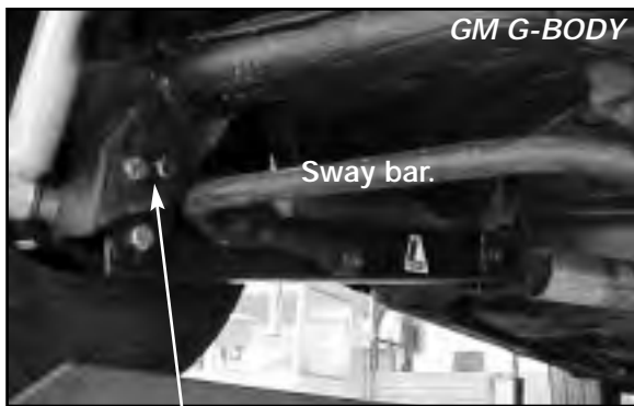
2 bolts here if not welding.
