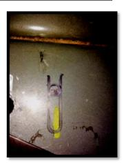
**Step 8:** Remove clip. Use a ½" drill bit and drill out the center mark. Slide the 3/8 clip back into position so the threaded part is aligned with the hole.
