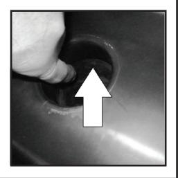
**57**- Apply extra sealant to top of grommets.
