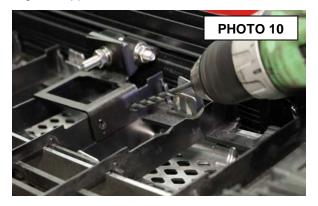
Secure bracket to grills using supplied button head Allen bolts, flat washers, and lock nuts. See Photo 11.
